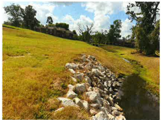
Rip Rap Repair
